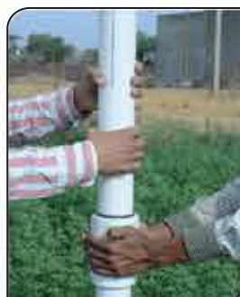
Hold Coupler before Loosening or Tightening of Pipes
